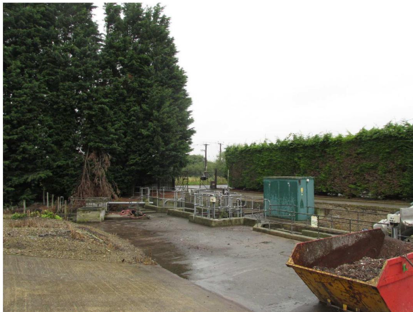
Figure 2. Photograph of application site.
