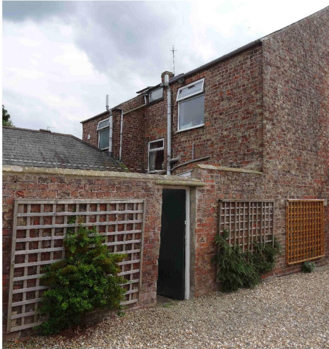
Fig 1.2 – View of rear from Westlea cottage drive
